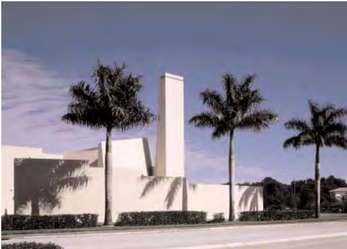
Top and above: South elevation. Photos by Rabinowitz Photography.
