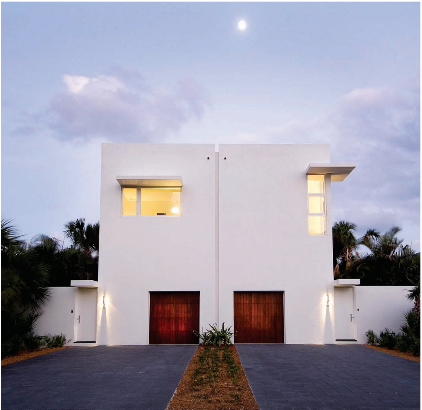
Main elevation. Note the use of fenestration to give the units individuality. All photos by Jerry Rabinowitz.
